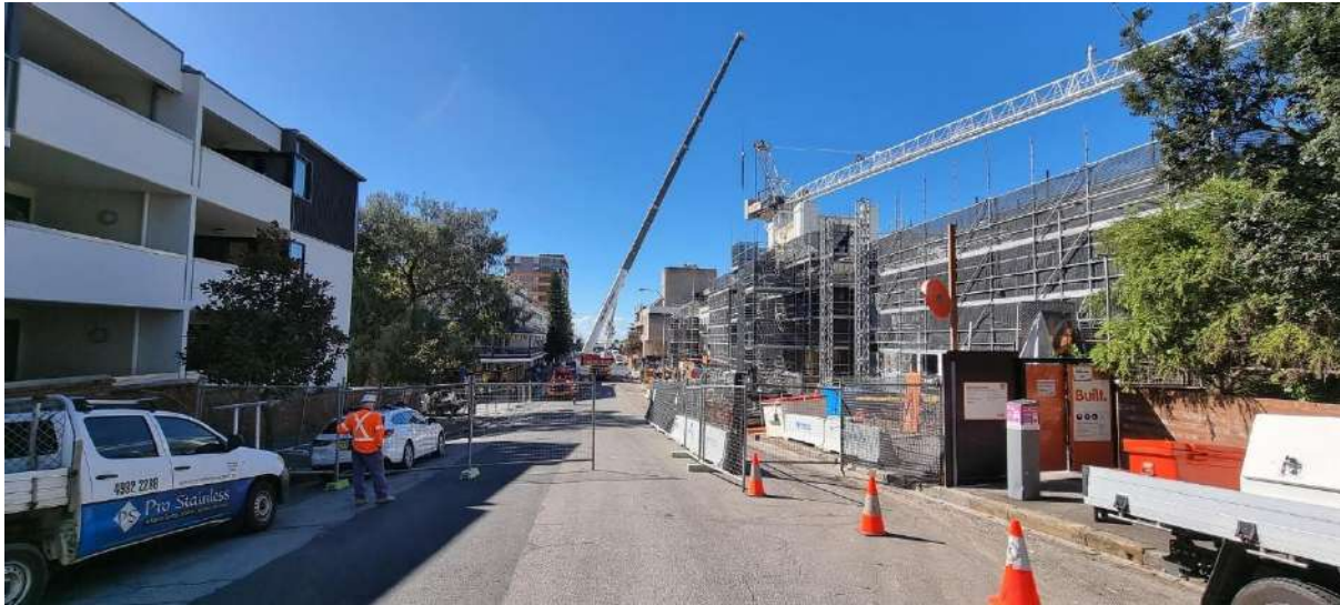
Photo 141: Tower crane dismantle
